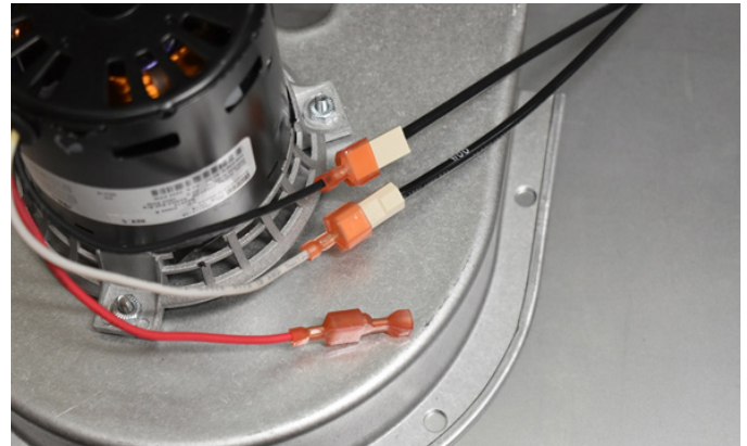
Figure 8: Factory Installed Inducer Motor Wiring
